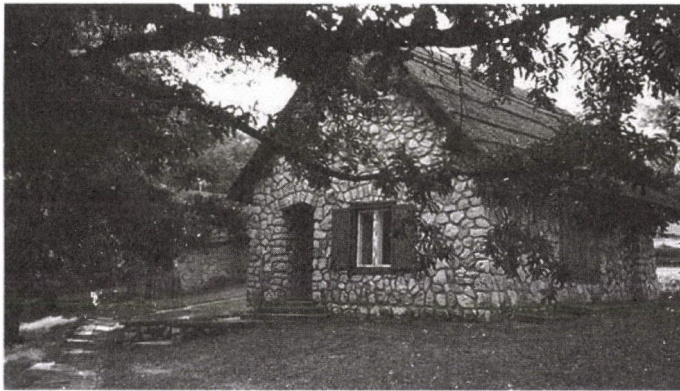
Fig. 3. The house for the measurement of the absolute values of the geomagnetic components (absolute house)
